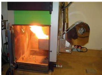
The 25kW Uni-Max burner during combustion
