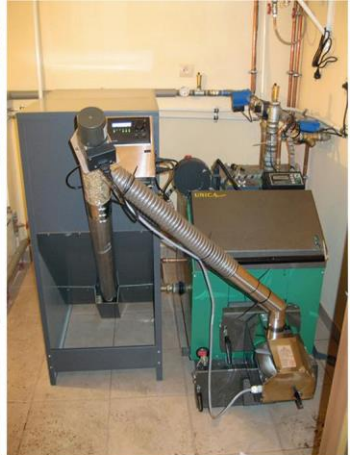
The Moderator-Unica solid fuel boiler with a 25kW Uni-burner
