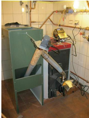
The Viadrus solid fuel boiler with a 25kW Uni-burner
