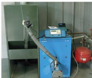
The Buderus oil boiler with a 32 kW Uni-burner
