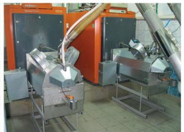
Viessmann Simplex boilers with 300kW Uni-Max Perfect burners
