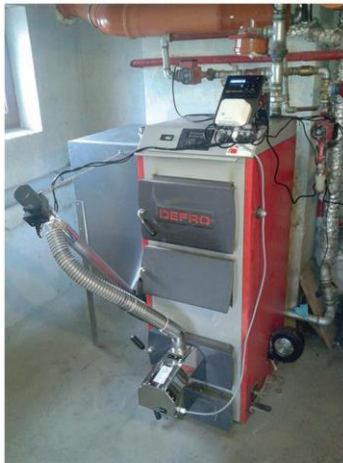
The Defro solid fuel boiler with a 25 kW Uni-burner
