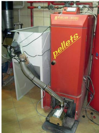
The Kiehar solid fuel chimney with a 32 kW Uni-burner
