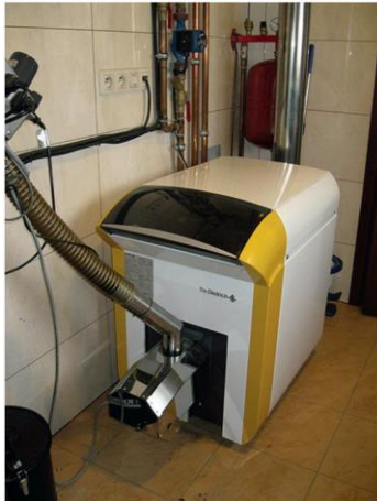
The Dietrich oil boiler with a 25 kW Uni-burner
