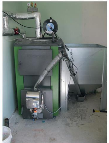
The Kamen Boiler with a 25kW Uni-Max burner
